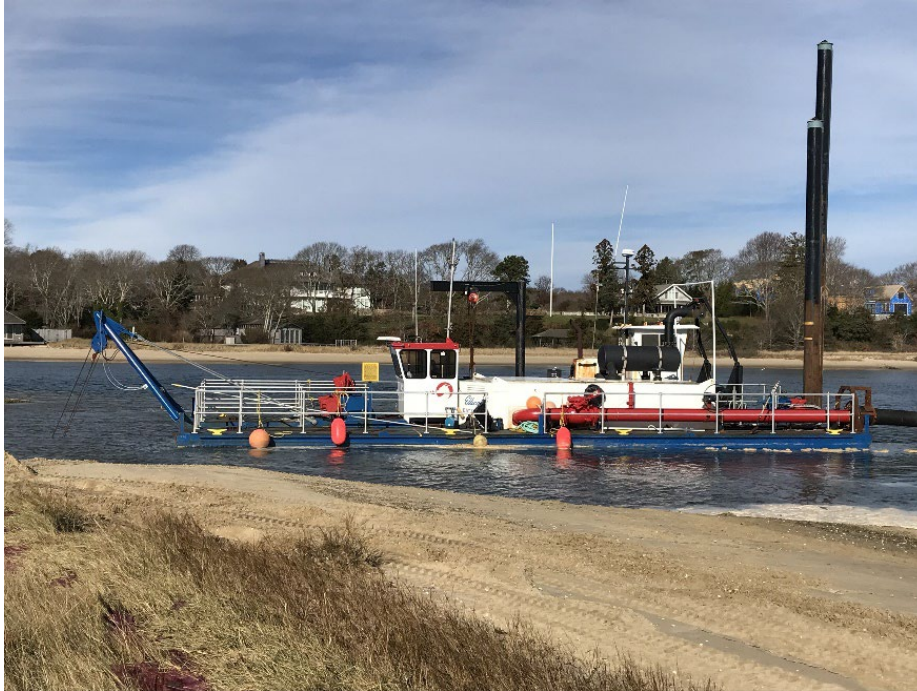
Figure 5-6: Hydraulic Dredging (Ellicott Dredges)
