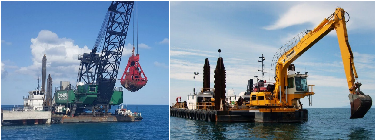
Figure 5-5: Mechanical Dredging – Clamshell (Cashman) and Backhoe (Seatools)
